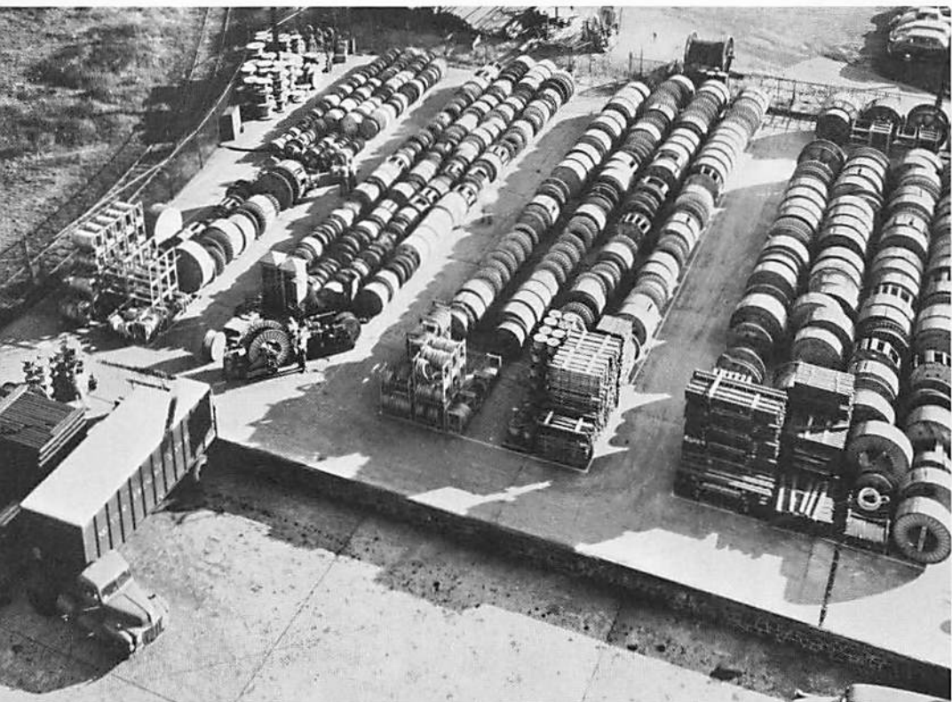
Cable and wire stored for the telephone company form an orderly pattern in cable yard of Distributing House.
