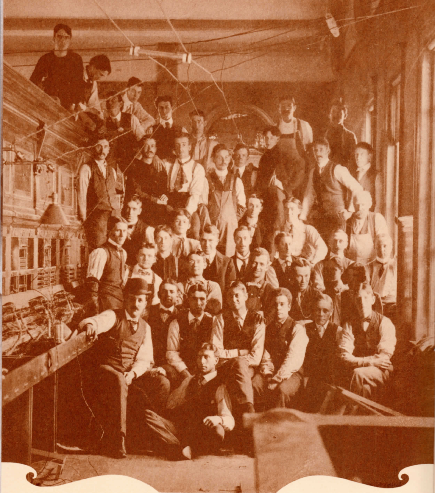
Switchboard installation in Oregon, 1900.
