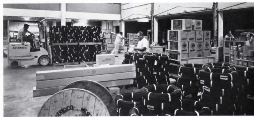
The year is 1964. Hurricane Cleo and, later, her equally destructive sisters Dora and Hilda played havoc with people, property and telephone systems. The Miami Distributing House (left) was just one of the many WE facilities that stayed open around the clock to ship equipment to disaster areas.
