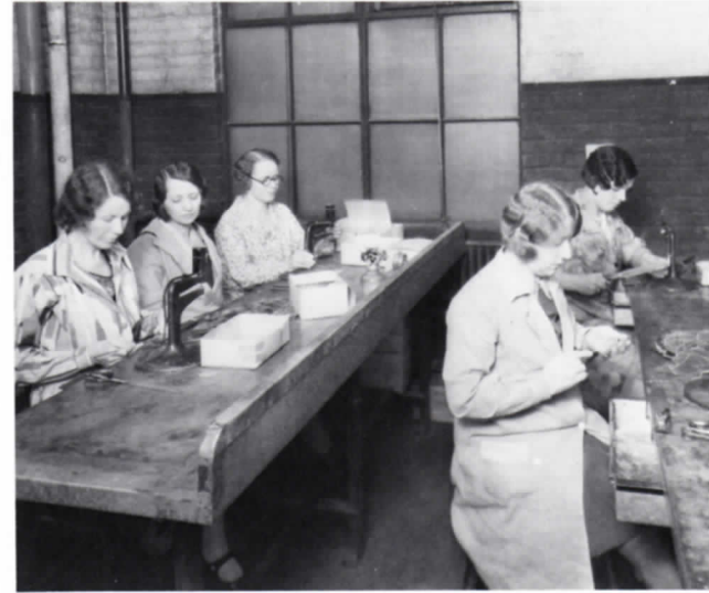
The early 30s —These women are testing sheets of mica that will be used to make capacitors. They were called condensers then. Electronic technology was well under way.
