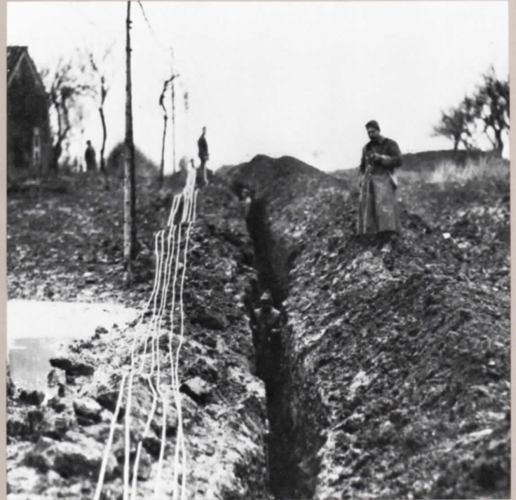
Trenches and World War I go together. This one near Ausauville, France, was for telephone cable. Like many during the war it was dug under continuous German battery gun fire. The date on this is 1918.
