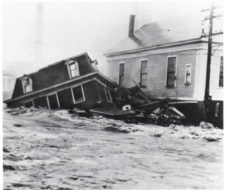
Floods again. This time, the scene is New England, where a hurricane swept central offices away in towns like Ware, Mass., above, and halted service for some 515,000 telephones. Repair crews from as far away as Southwestern Bell territory were mobilized to deal with the emergency and get things back to normal. The year was 1938.
