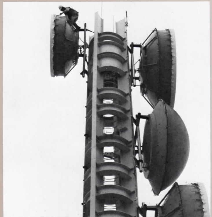
Below—Digital transmission systems were an increasingly important part of the network in the 70s. This unusual tower in Eugene, Oregon, was part of the first DR-6 digital system.
