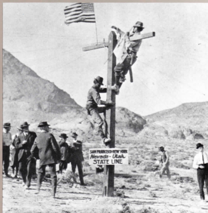
June 17, 1914: The final pole of the first transcontinental telephone line is put into place on the Nevada-Utah border. A great push was made to complete the line in time for the opening of the Panama-Pacific Exposition, only to have the opening postponed a year.
