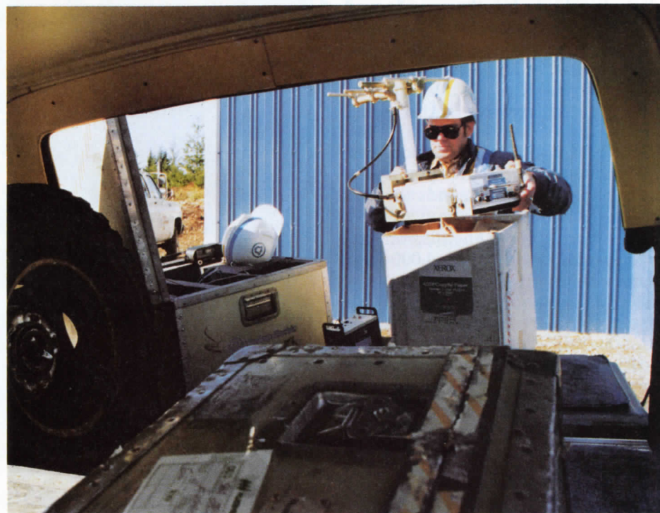
Above—Bob Herring from the Denver Turnkey group unloads radio gear at West Harness. Left—he directs the antenna crew working on the tower.
