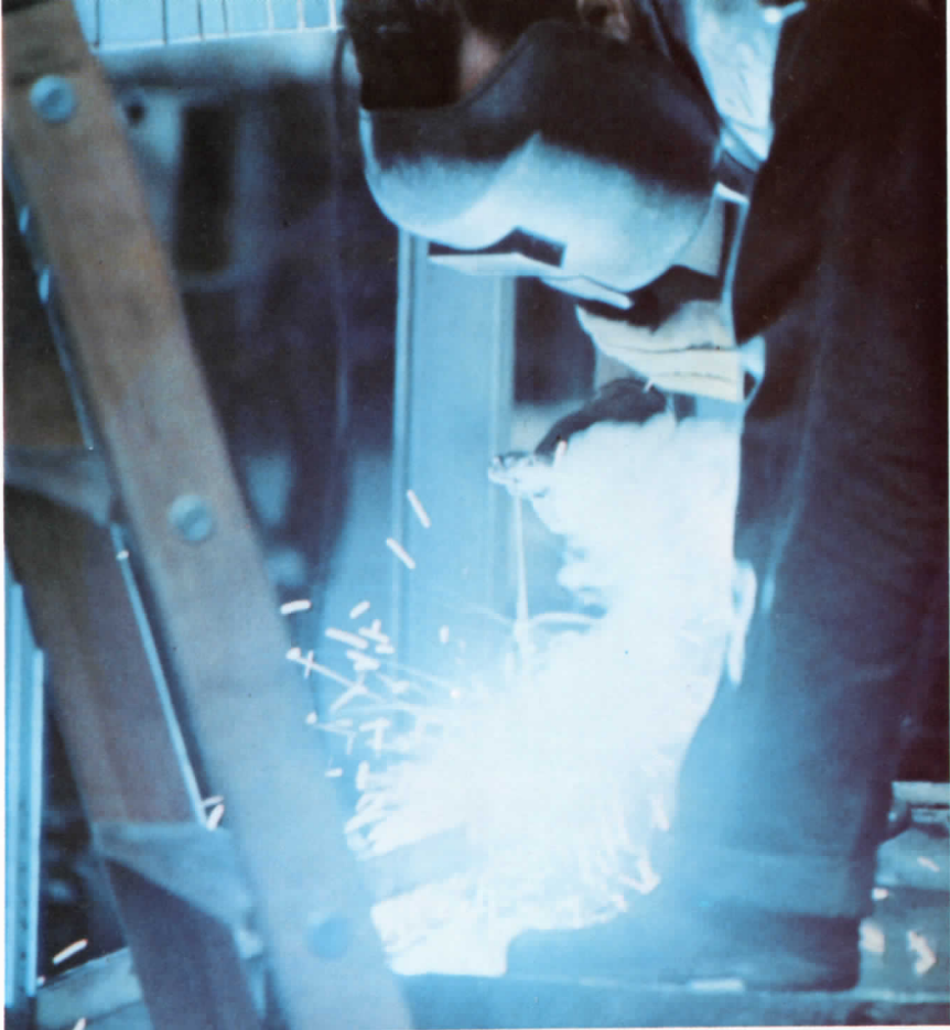
One of the responsibilities of the Works Service organization is to make weld modifications in manufacturing areas to accommodate equipment.
