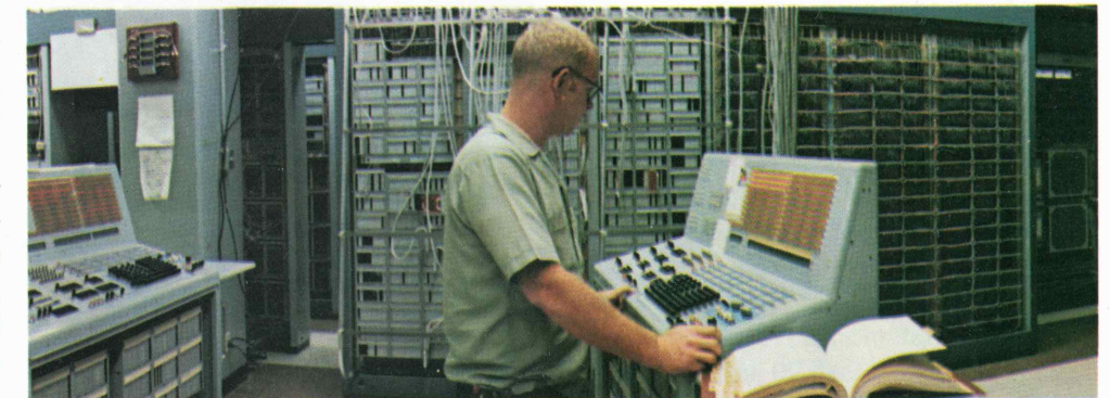
Top: WE personnel install the first of a new frame system called Cosmic-Cosmos at the Beverly Hills central office. The new system helps maintain order in the maze of wires coming into a central office and helps the telephone companies realize savings in both wiring and clerical costs.
