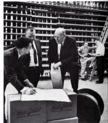
WE equipment engineers review plans with a Bell Telephone Company engineer at a central office installation.
