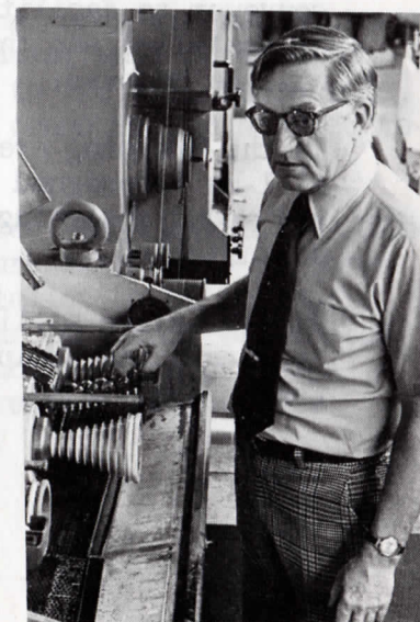
CABLE AND WIRE PRODUCTS: Above - Joe Swenson checks the cable lay at the Northampton strander take-up. Bottom left - Bill Kinsley examines the edge-forming key in steel tape overlap die. Bottom right - Lee Baldauf checks the die string-up on SAMP No. 4 wire drawing machine.
