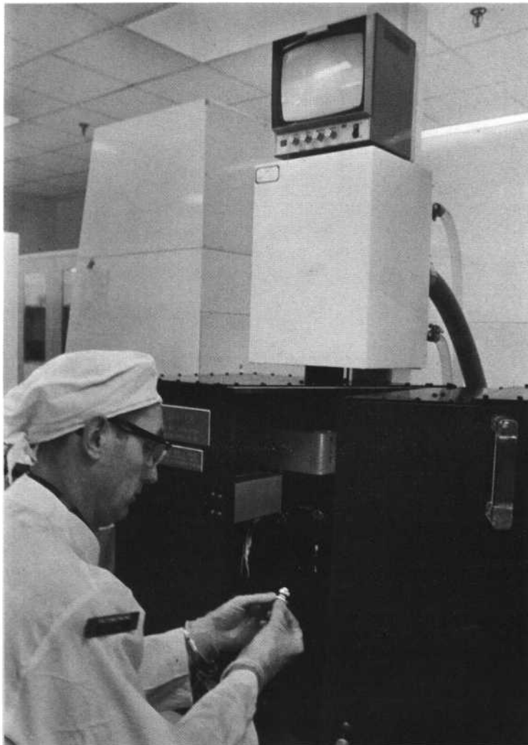
A pulsed ruby laser inside this "black box" ensures precise alignment of the camera tube's beam-stripper—the electrode that trims the electron beam to a diameter of 0.003 inch. After the beam stripper is aligned with other electrodes, the laser bores a 0.003-inch hole through it. Bob Sell, on assignment to the Reading Laboratory from the Western Electric Company, is shown loading an electron-gun structure into the unit. He will use the television monitor to aim the beam.
