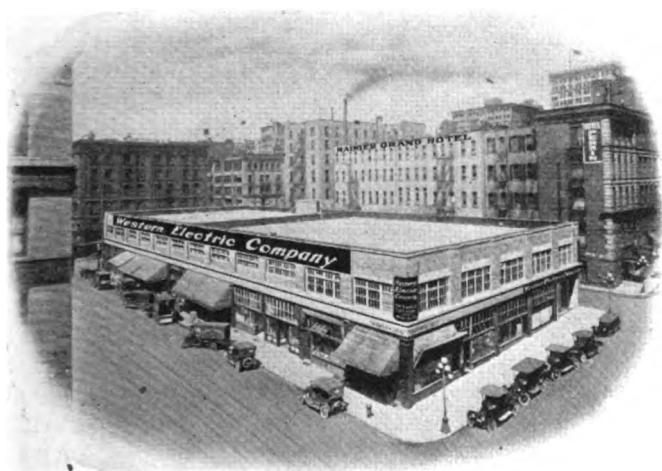
Seattle's New Location
