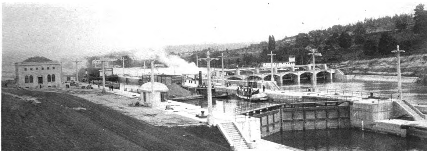
General View of Locks Showing Administration Building to the Left. The Lighting Standards are Unique but Very Effective
