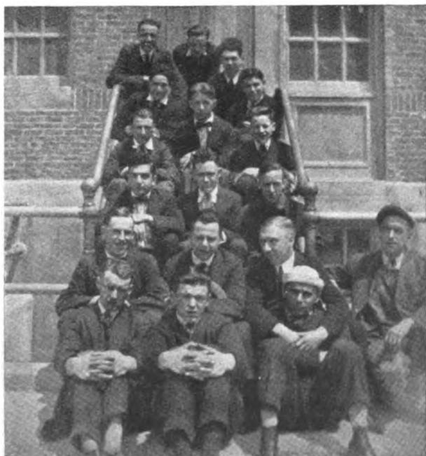
M. Shannohoffski Sends the NEWS This Picture of Installers on the Gloucester, Mass., Job. Who Subscribed $1,000 to the Liberty Loan After a Rapid-Fire Canvass by Foreman C. L. Priest
