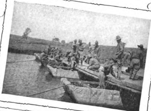
BUILDING A LIGHT PONTOON BRIDGE
