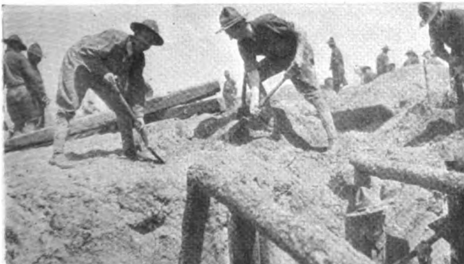
Our Two San Francisco Rookies Working in Construction of Bomb Proof Shelter of Trenches at Monterey, Calif.
