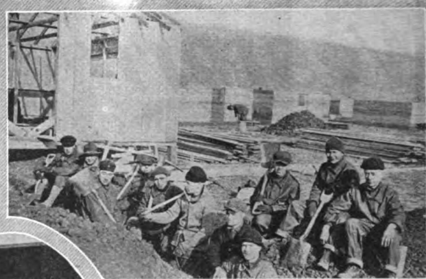
Some of the Hawthorne Boys Helping to Build the Medical Detention Camp
