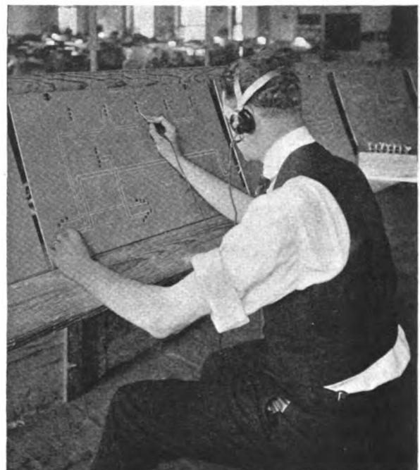
Student Learning to Trace Continuity of a Standard Circuit. These Boards Are Wired on the Back to Reproduce True and False Electrical Conditions at Various Test Points
