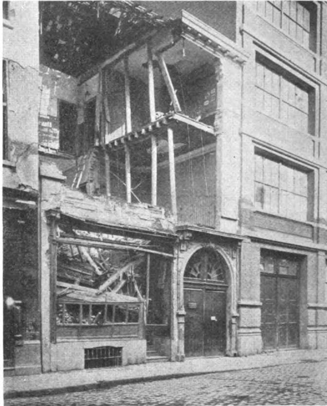
A Shot That Came Too Close for Comfort. The Building on the Right Is Part of the Antwerp Factory
