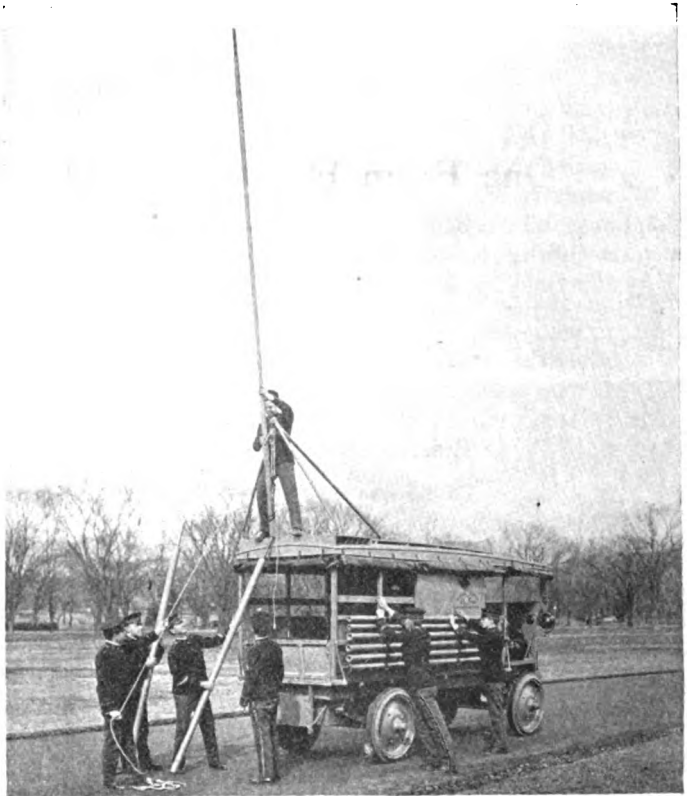
Erecting the Mast for a Tractor Set—Wireless Telegraph
