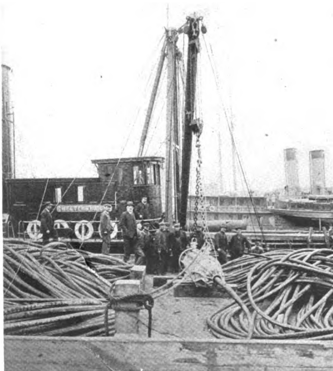
The 16,000-pound Strand Run from Shackle at the Top of the Sling and Fastened to Cable to Ease the Strain Near the Loading Pot When Lowered Into the Water
