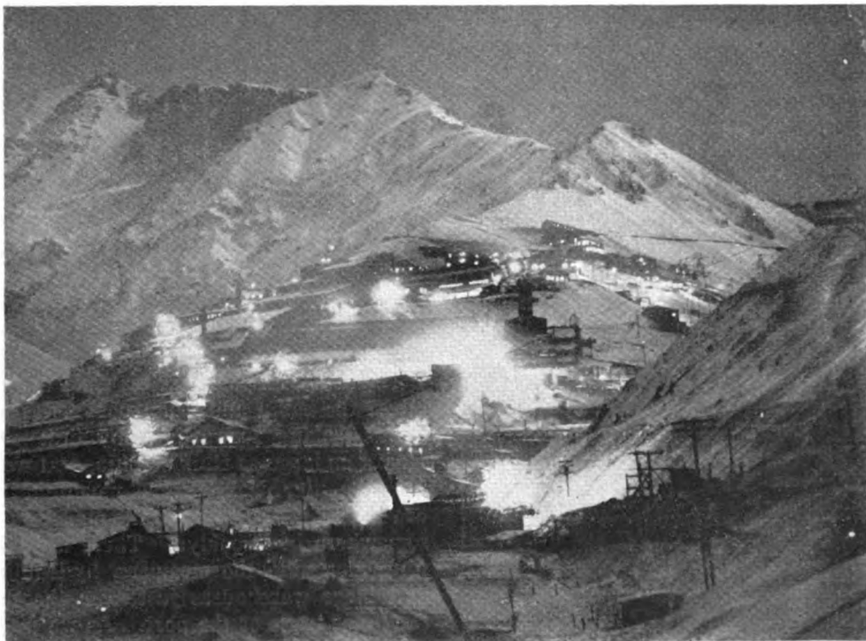
A Night View of the Same Mine Shown on the Front Cover. By Night, Braden is a Great Flare of Electric Light
