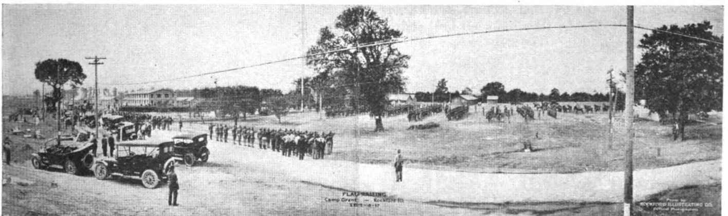
The Cable in the Upper Part of the Picture Doesn't Add to the Artistic Effect, But it Does Prove That the Western Electric Installers Had Been on the Job Before This Flag-Raising Took Place at Camp Grant
