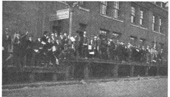
Ready to Leave the Building
