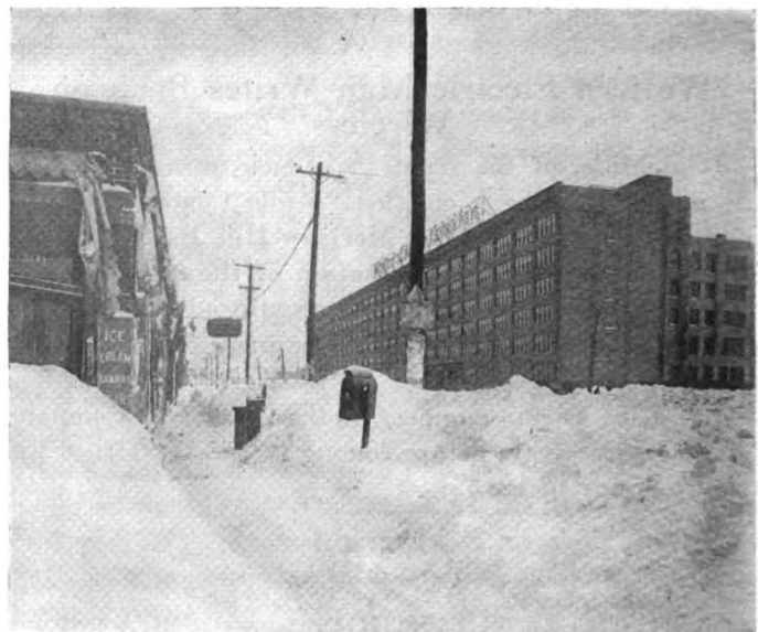
Twenty-second Street Looking Toward T. A. Building. Somewhere in the Drift to the Right is a Motor Truck Completely Buried
