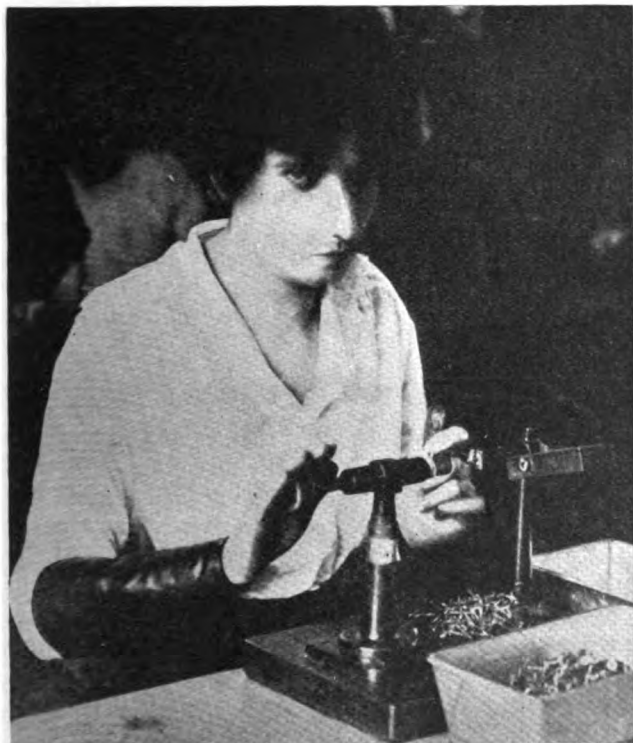
Fig. 3—Assembling the Coil in the Shell
