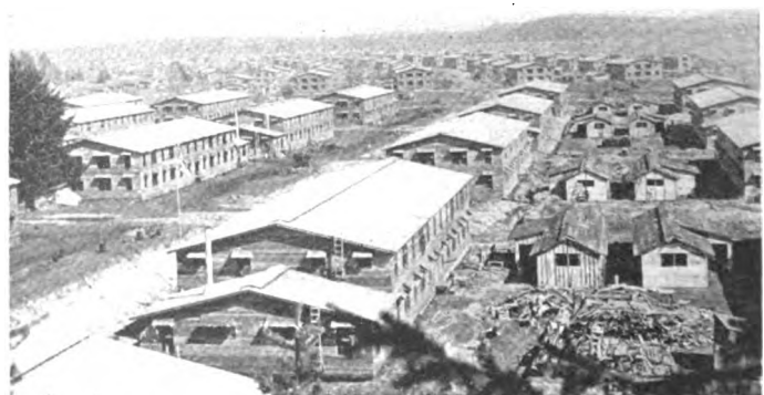
Cantonment at American Lake, Wash., Under Construction
