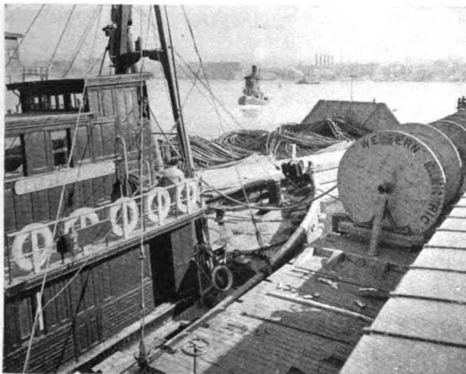
How the Reels Were Jacked Up and Braced in the Laying of the Tarrytown-Nyack Cable
