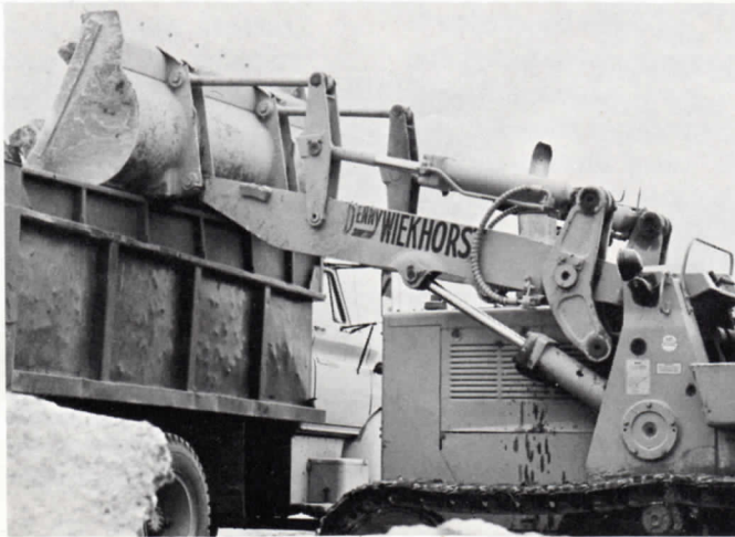
The old concrete is removed to make way for a new surface.
