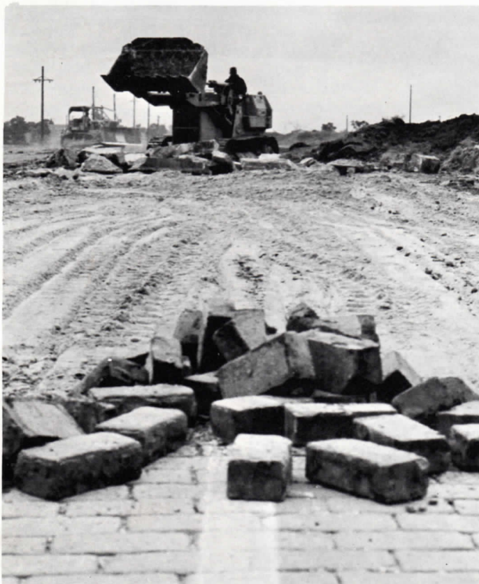
The old cobblestone street gives way to a modern four-lane street running from West Center Road to "L" Street.
