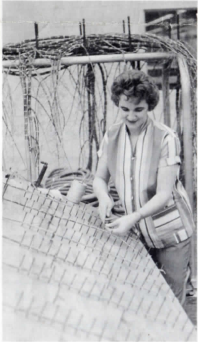
After forming a cable, Cecilia Schultz skins insulation off 24-gauge wires.
