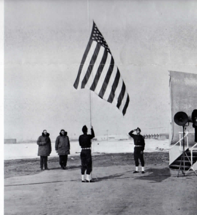
Members of the Omaha Works'-sponsored Explorer Scout troupe raise the national colors opening the ground-breaking ceremony.
