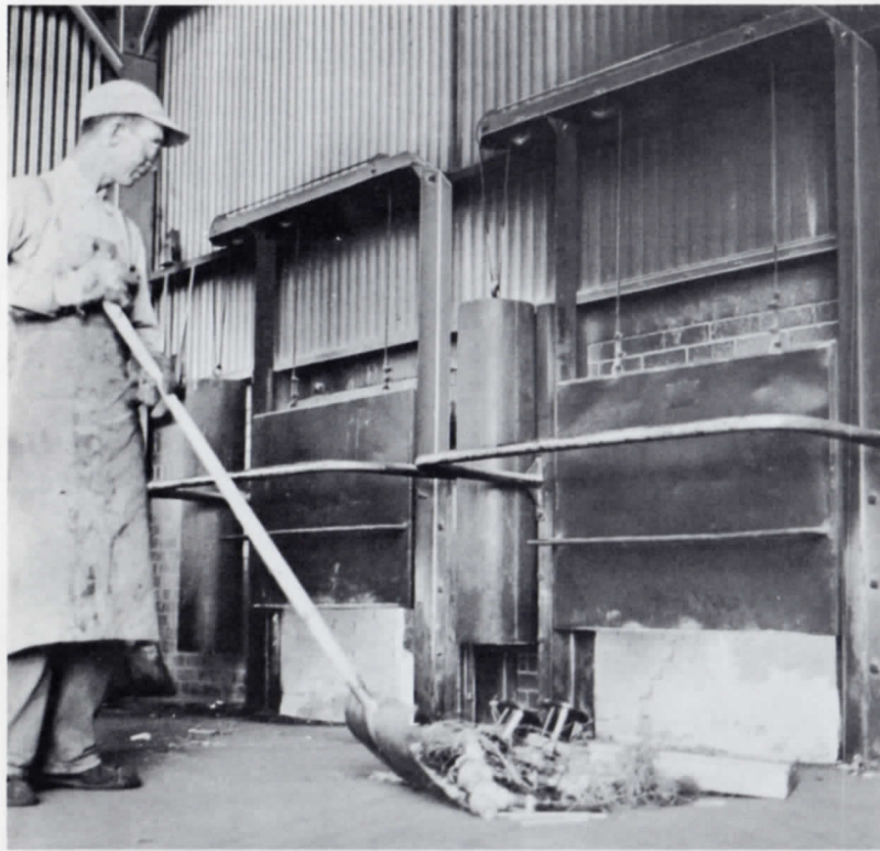
Paul Ryan (271) shows what would have happened to salvable materials had they not been sorted from rubble.
