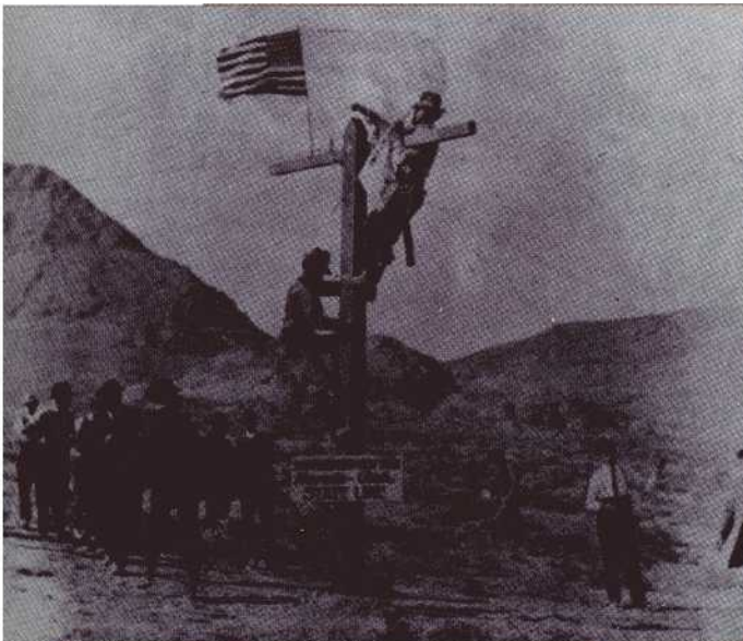
The lead-sheathed cable these linemen are installing, above, circa 1900, would reduce and virtually eliminate the use of open wire for aerial telephone lines.
